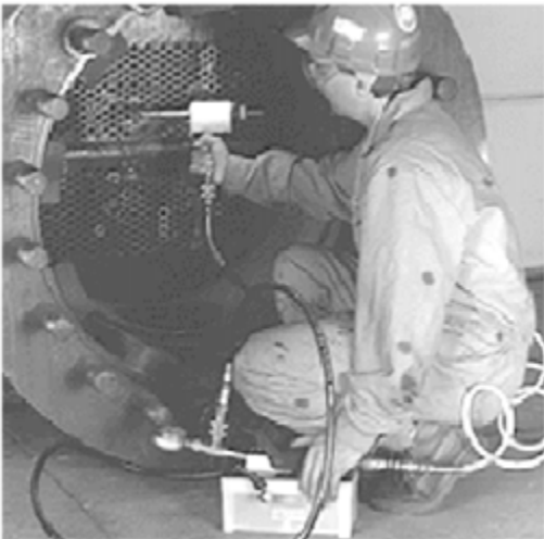
Figure 312-4.2-3 Typical Installation of Mechanical Fit Tube Plugs
